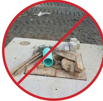
2. Final paving must be completed. Final paving ensures that paving materials will not enter and contaminate the Filterra HC system during the paving process, and that the plant will receive runoff from the drainage area, assisting with plant survival for the Filterra HC system.
