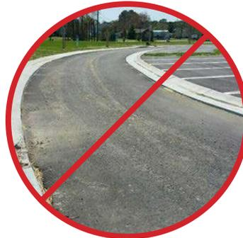
3. Filterra HC throat opening (if applicable) should be at least 4" in order to ensure adequate capacity for inflow and debris.
